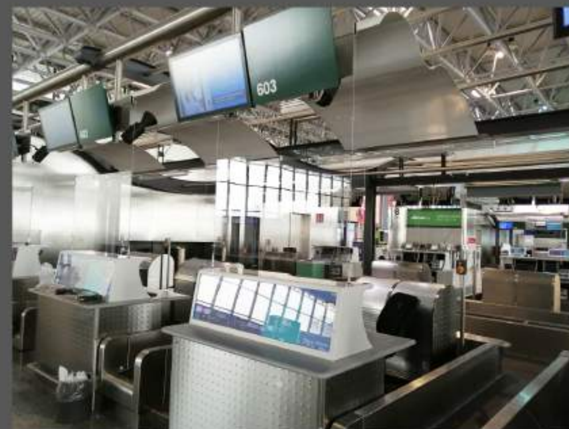
Installation of two 93x80 cm methacrylate panels.
